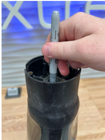
Figure 2: Marking Drilling Location
